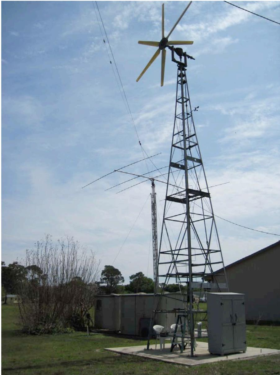
Figure 1. The completed wind generator. Note the anemometer and wind vane near the top of the tower and the narrow shaft inside the right section of the tower that turns the turbine section into or out of the wind.
