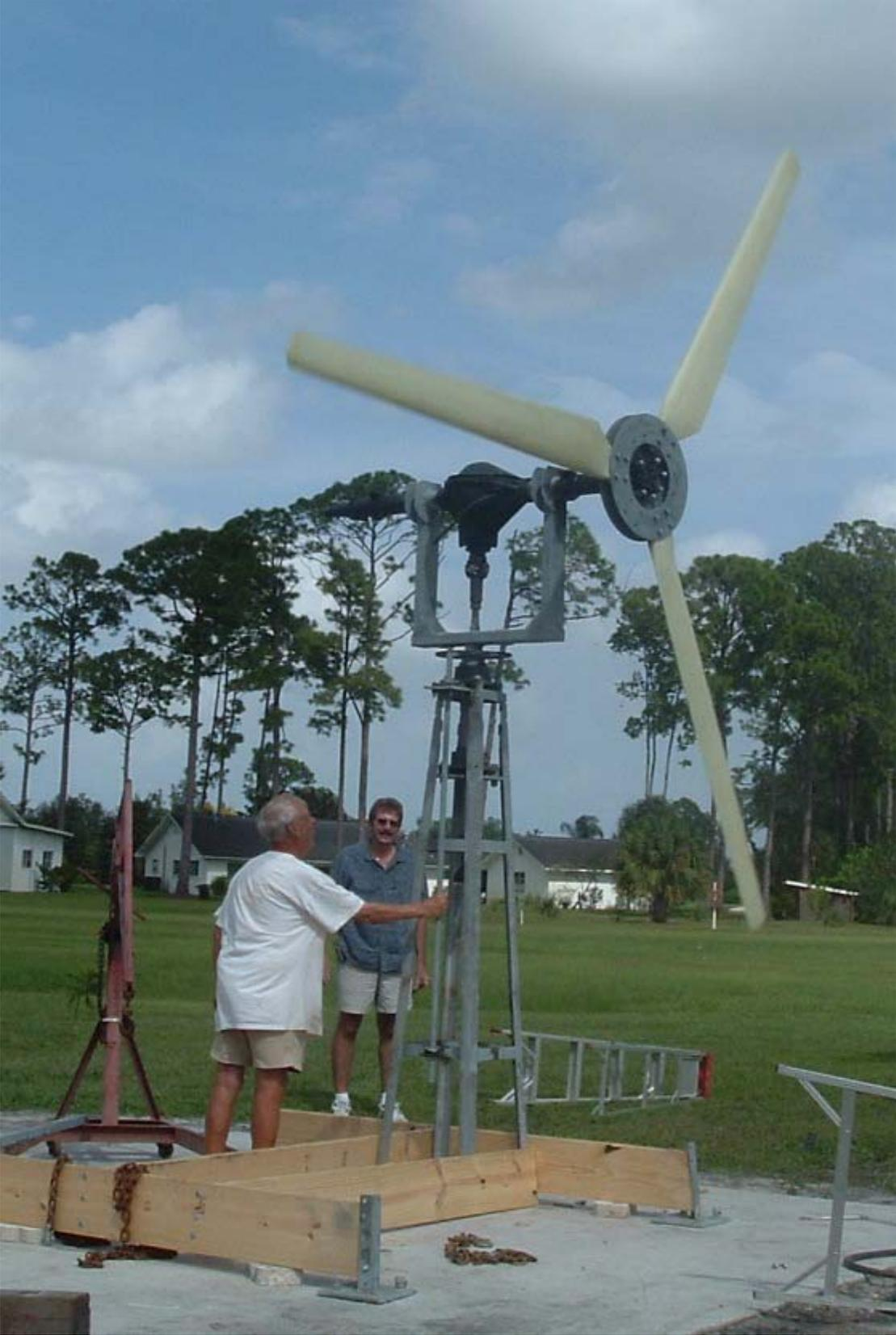
Figure 4. A close-up view of the tower top. Note the mounting of the truck differential. A large gear mounted underneath the U-shaped bracket will turn the turbine into or out of the wind.
