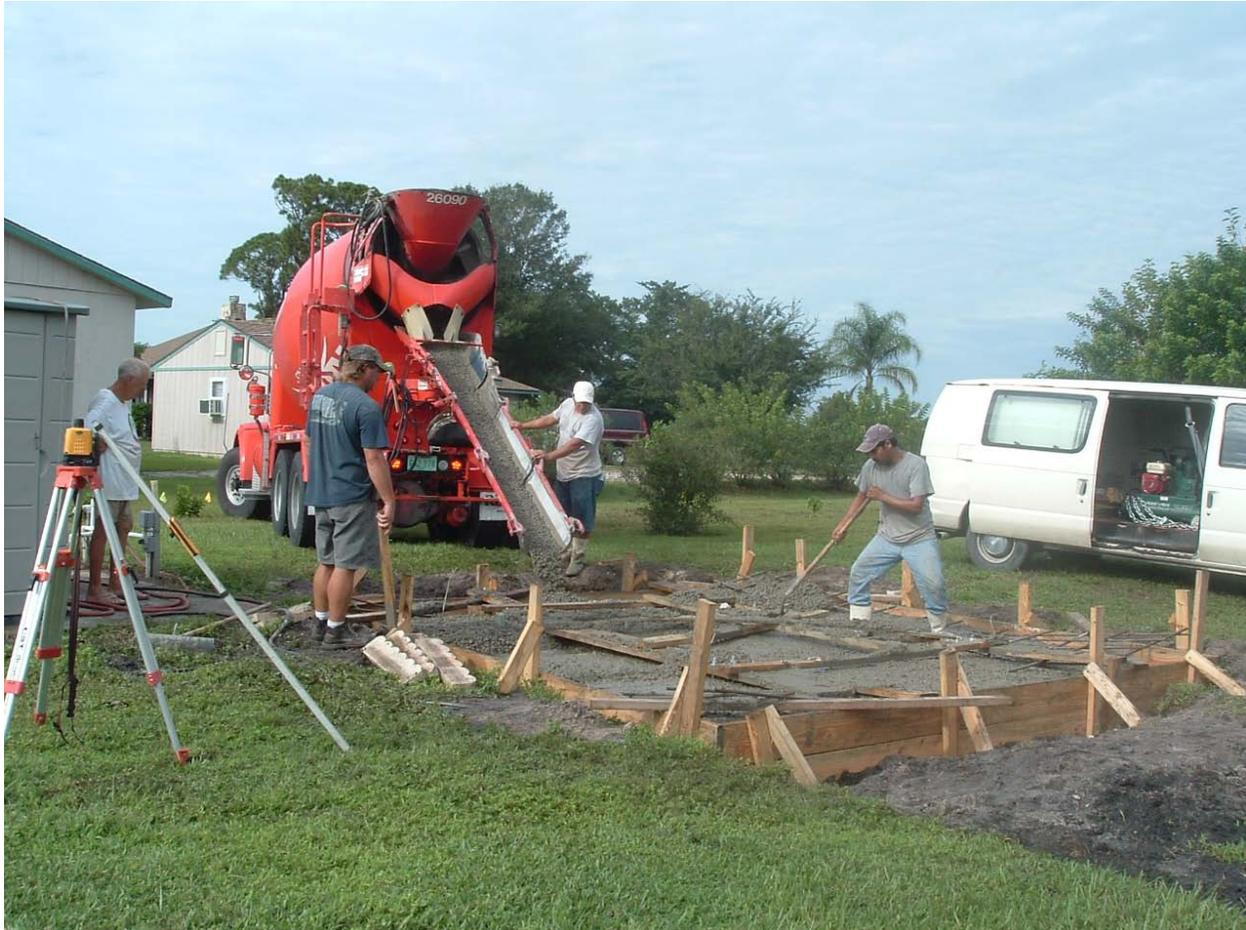
Figure 2. Pouring concrete for the engineered base.
